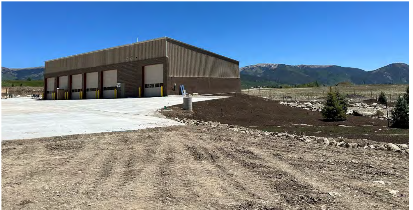
6. Grading, Landscape, and Concrete Completed at the Rear of the Property.
