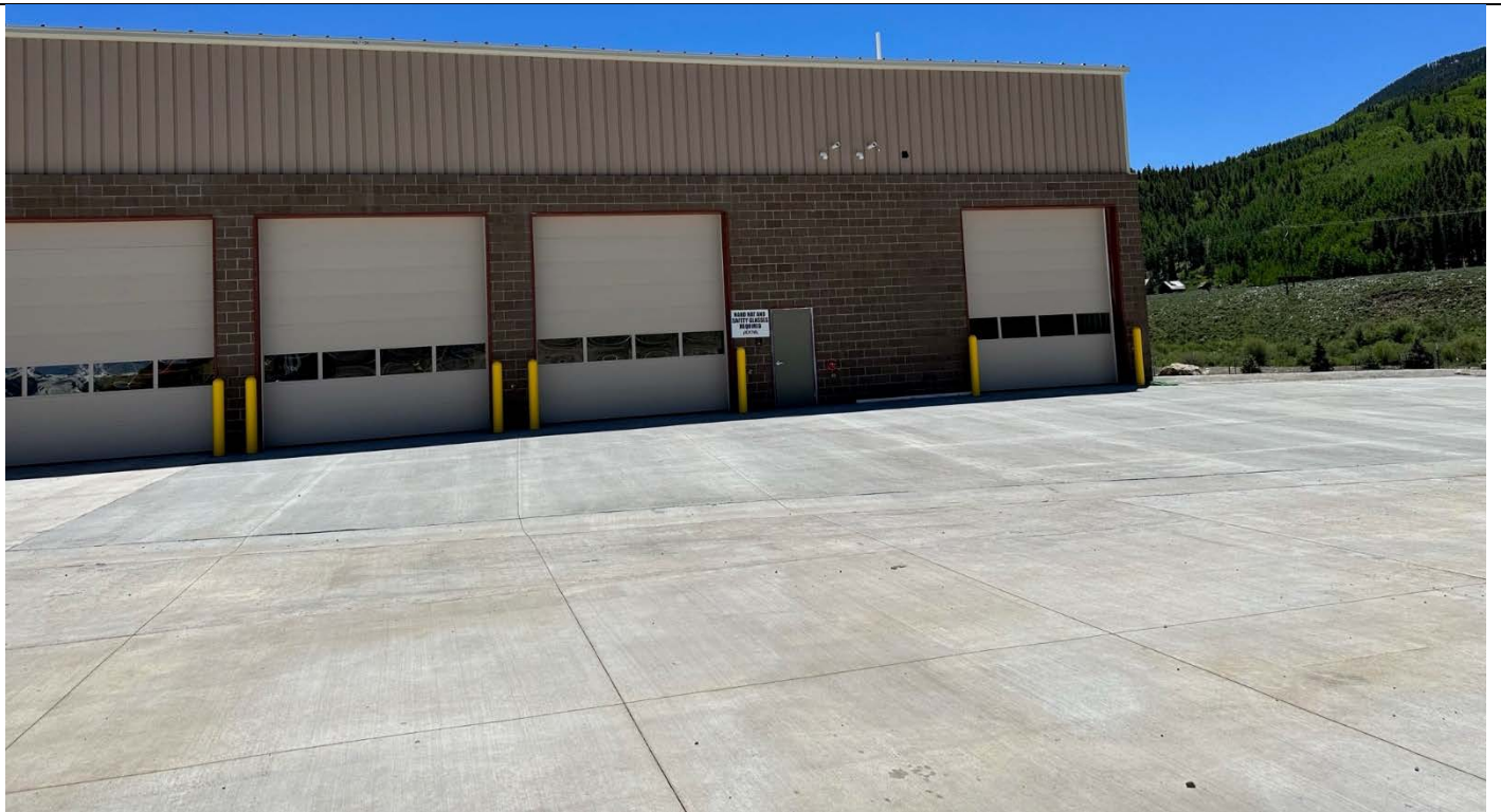
5. Remaining Exterior Concrete Poured.
