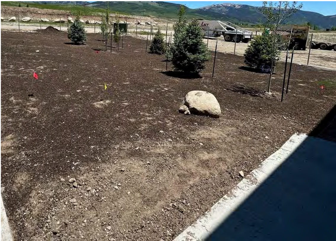
1. Front Landscaping and Sidewalk Placed.
