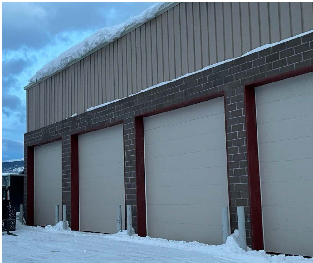
3. Sectional Garage Doors Installed in All Six Bays.
