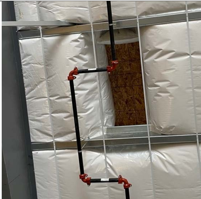
2. Roof Curbs for Air Handlers Installed.
