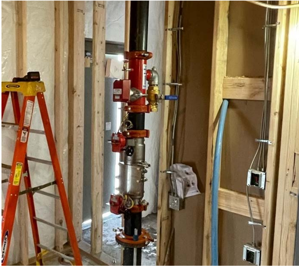
1. Fire Riser Assembled in Mechanical Room.
