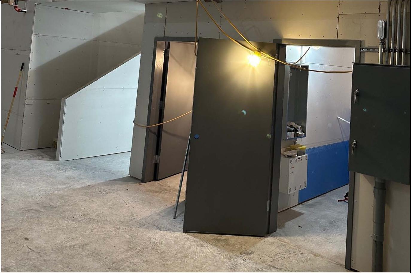
4. Drywall and Hollow Metal Doors Hung Outside Mechanical Room.
