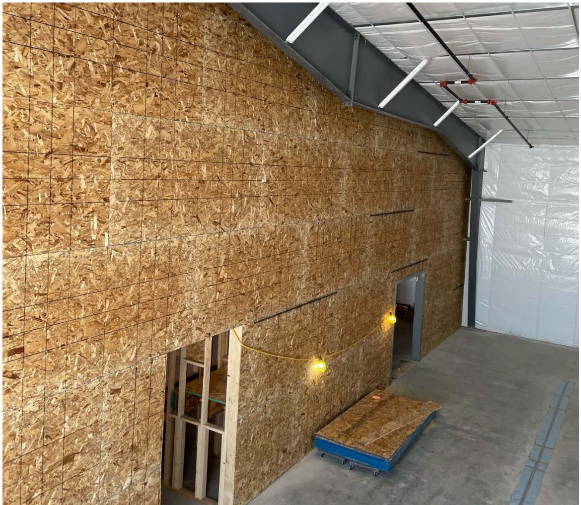
4. Mezzanine Wall Sheathing
